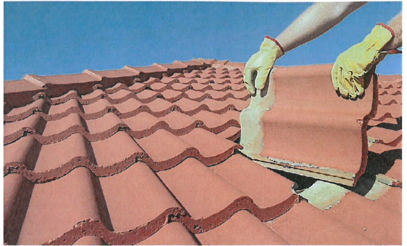
Know your rights when it comes to construction contracts.
